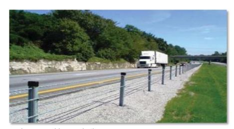
Photo 6: Cable Guardrail
