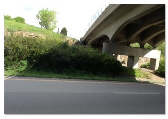
Photo 3: Pier protection that does not meet standards
